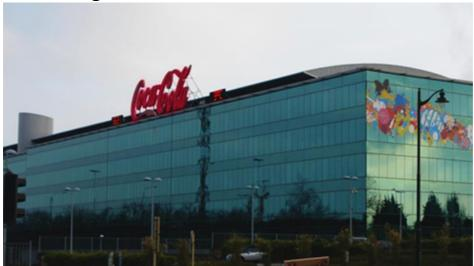
The existing windows in the Coca-Cola® Building in Brussels are double glazed. To improve the solar gain value (g-value) a total of 1.660m² Umiscreen coated IR films were installed on the 510 windows for the price of 99.576 €. This glazing retrofit creates a profit of 14 €/m²/year.
